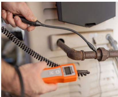
Inspecting a gas pool heating system
